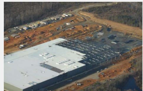
Lidl Distribution Facility, Spotsylvania County
