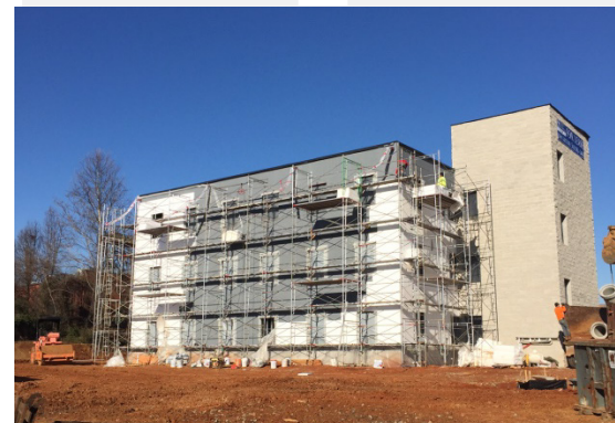
New 12,000 SF, 3-Story Office, Spotsylvania, VA
